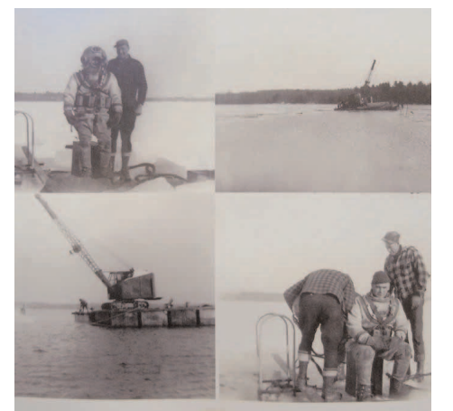
Kent London's series of photos show divers replacing an intake pipe for Kennebec Water District in 1952.
